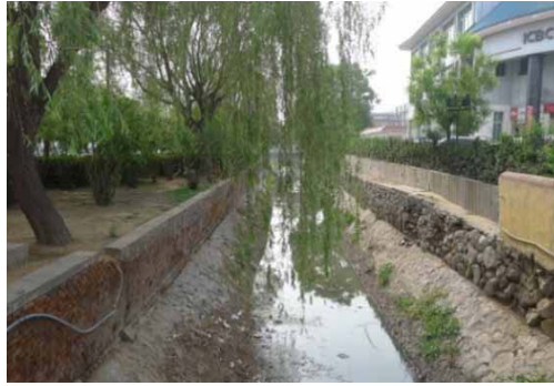
Figure 1. Low water system landscape (Source: Internet search and collation).
