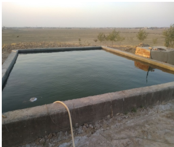
Figure 1. Concrete pool for watering.
