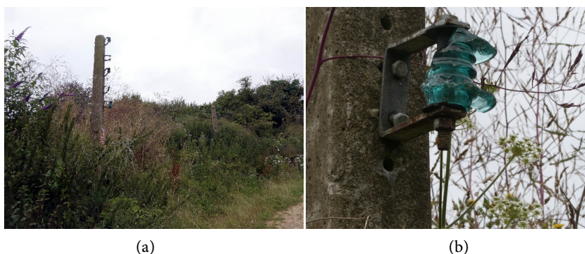
Figure 8. electrified protection barrier—(a) Remains of two concrete supports; (b) Glass insulation element, details.
