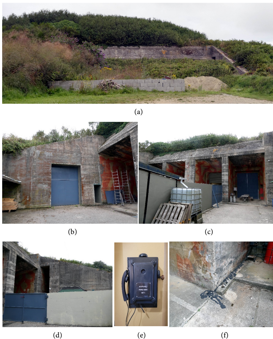
Figure 4. Reinforced, buried bunker—(a) Coverage three meters thick; (b) Entrances of the electrical power plant; (c) Entrance square and four garage cells for special vehicles with orange camouflage; (d) Entrance of the rooms and depots for the troop; (f) Internal telephone; (g) Watertight insulation.
