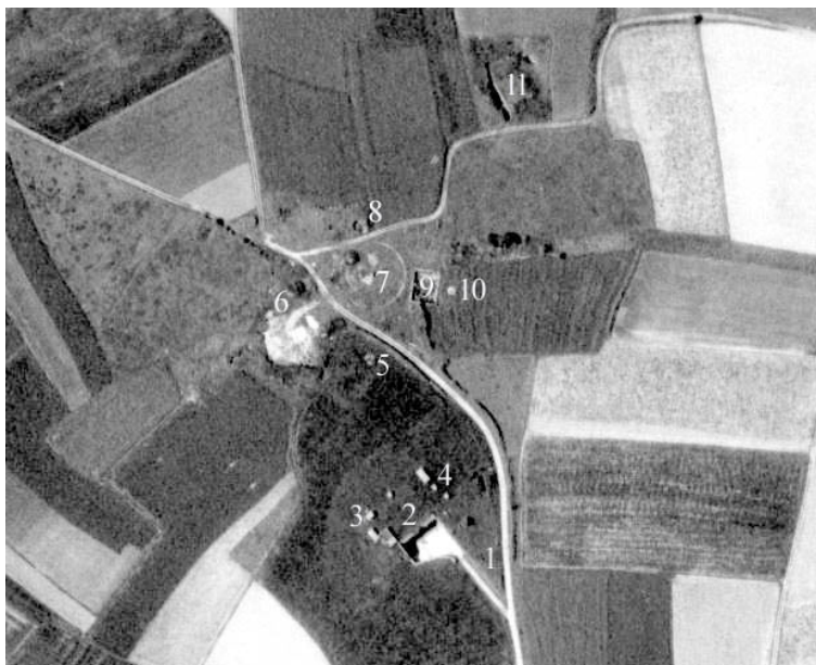
Figure 3. radio guidance station K11, Stp Mo 44c of Saint-Fiacre—1, tobruck; 2, reinforced, buried bunker; 3, concrete barracks or ventilation towers; 4, three concrete barracks or ventilation towers; 5, possible light Flak emplacement or tobruck; 6, L409 Flak emplacement; 7, Knickebein single rail ring; 8, possible light Flak emplacement or tobruck; 9, pit for shack or cistern; 10, possible Flak emplacement or tobruck; 11, R622 . C0515-0021_1966_F0515-0915_0110, n° 110, ech. 1/23364, Argentine, 16/05/1966.
