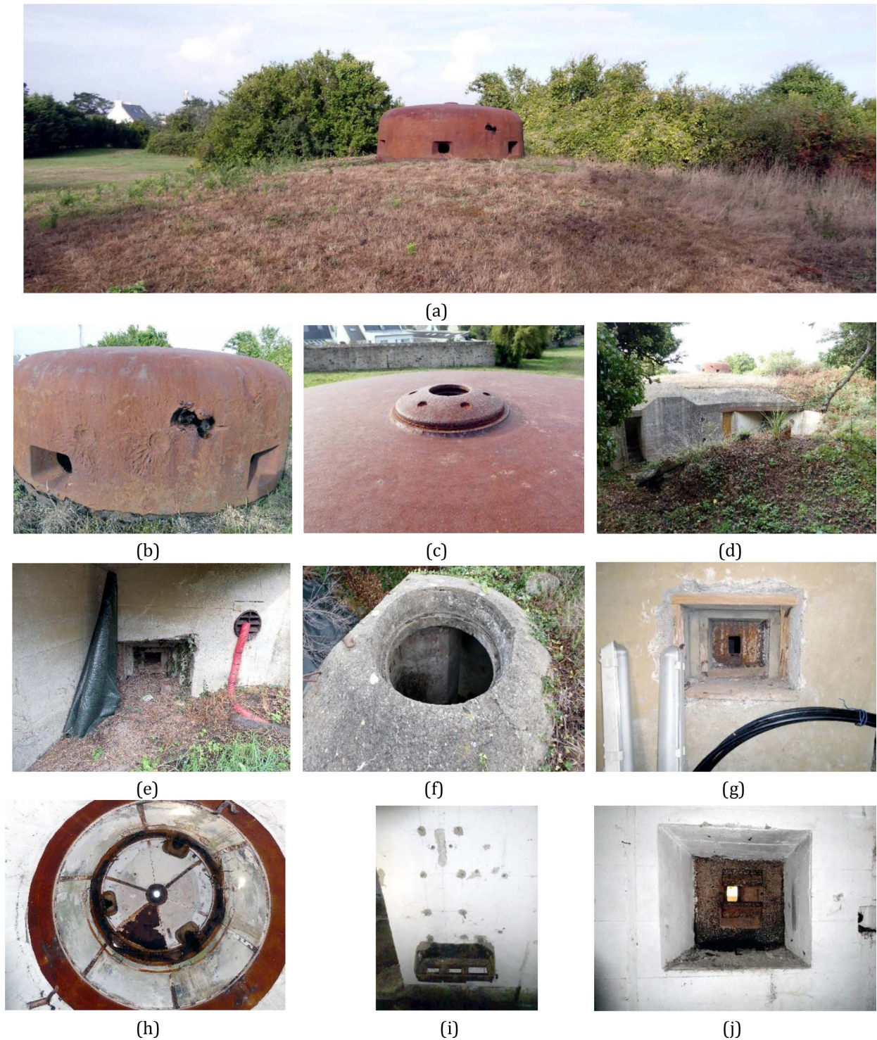
Figure 3. R 634 (15) : (a) General view; (b) Six embrasures cupola, external view; (c) Periscope opening; (d) Front side, on the left tobruck entrance; (e) External embrasure with splinters of the close combat room (3); (f) Tobruck opening; (g) Embrasure with splinters of the entrance; (h) Six embrasures cupola, internal view; (i) Support for telephonic connections; (j) Embrasure of the crew room.
