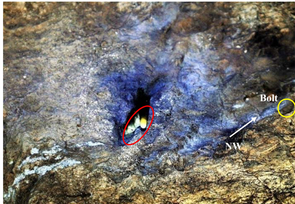
Figure 13. Zone 1 ceiling speleothem (rotated into the orientation as seen in Figure 11 ). We attribute the distinctive deep blue coloring (filter enhanced) to the presence of organic carbon compounds contributed from soot and calcified fibers embedded in plaster. Note the presence of what is now a kind of calcified bolt (encircled yellow) emplaced in the ceiling near the speleothem.
