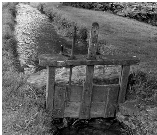
Figure 6. An ancient (Middle Ages) sluice gate crossing a village stream in Morland, Cumbria UK. Note the hand crank on the upper left of the frame. Source: https://lindamphotos.wordpress.com .
