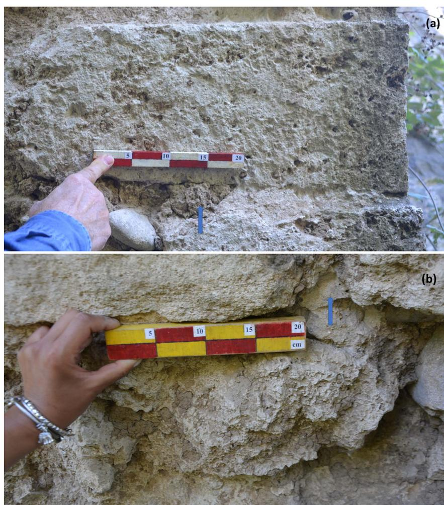
**Figure 10.** The phytoclastic travertine ashlars, showing the characteristic pores, and the mortar of arch 2 (a) and arch 3 (b), from which the samples PO 1 and PO 9, PO 2 and PO 10 were collected, respectively. The mortar is highlighted by arrow.
