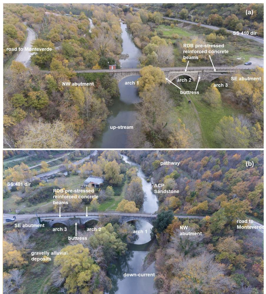
**Figure 6.** Current state of the façade of the POB as seen through the drone up-stream (southwest) in (a) and down-stream (northeast) in (b). The abutments, the arches 2 and 3 and the cutwaters are covered by weed and climbing vegetation. The pathway in (b) coincides with the layout of the old Appian Way.
