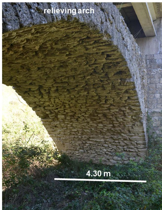
**Figure 8.** Face of the arch 3, 4.30 m wide, showing the *opus incertum*, consisting of marly and siliceous limestone pebbles with a blade shape and tiled structure, and the relieving arch with the squared ashlar of phytoclastic travertine.
