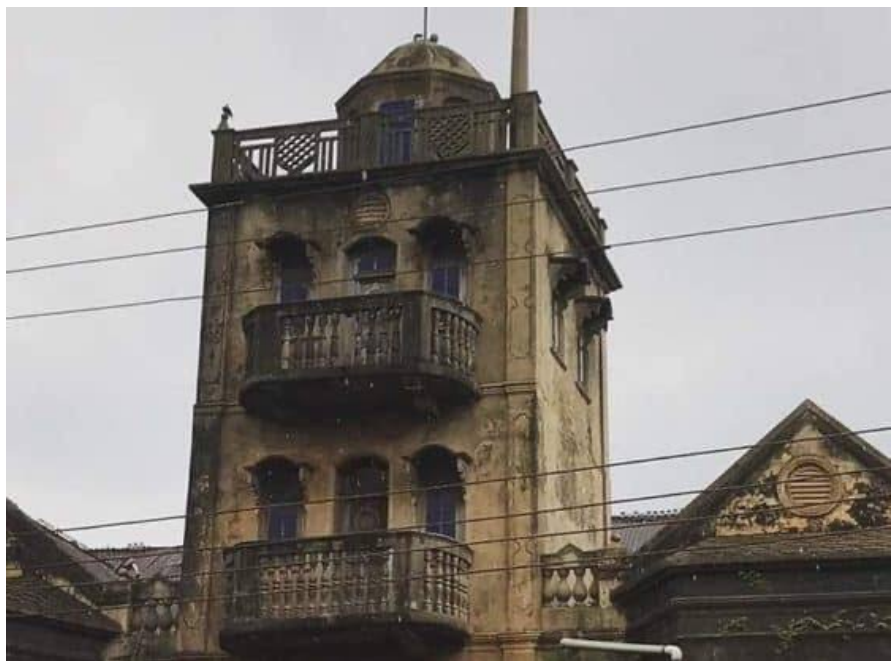
Figure 2. Building during the colonial era, during the first few stages of globalisation.
