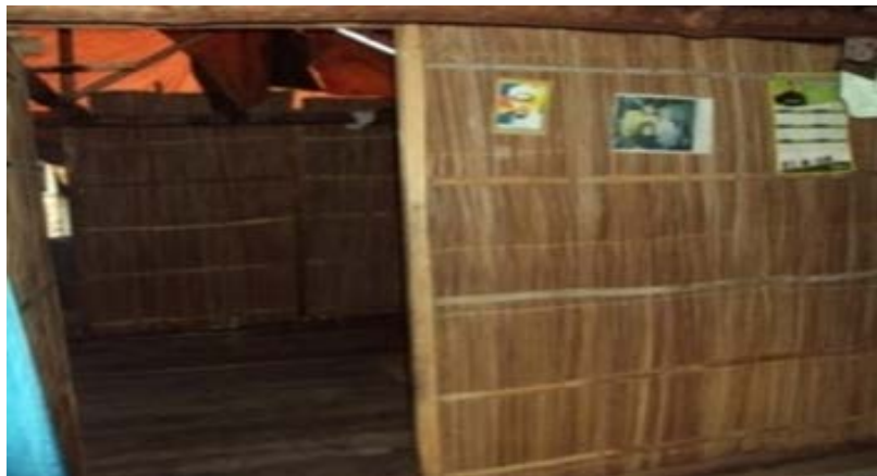
Figure 11. Building cover material the inside uses leaves weaved. Source: Researchers' recorded images in 2010.
