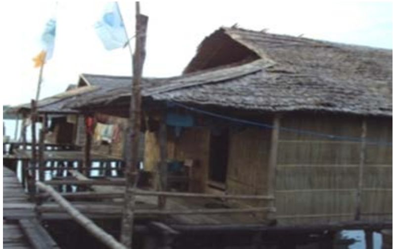
Figure 10. Building cover material from walls made from plaited leaves. Source: Researchers' recorded images in 2010.
