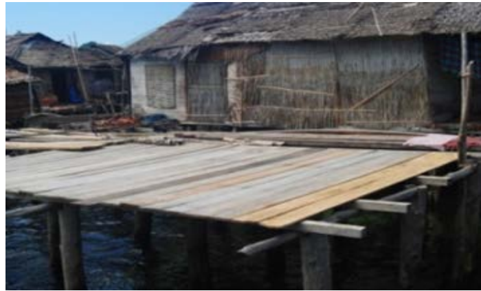
Figure 3. Pole and floor of Ruamah Bajo. Source: Researchers' recorded images in 2009.
