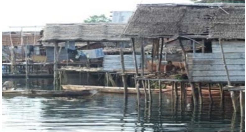
Figure 7. Buildings with continuous wooden frames. Source: Researchers' recorded images in 2009.
