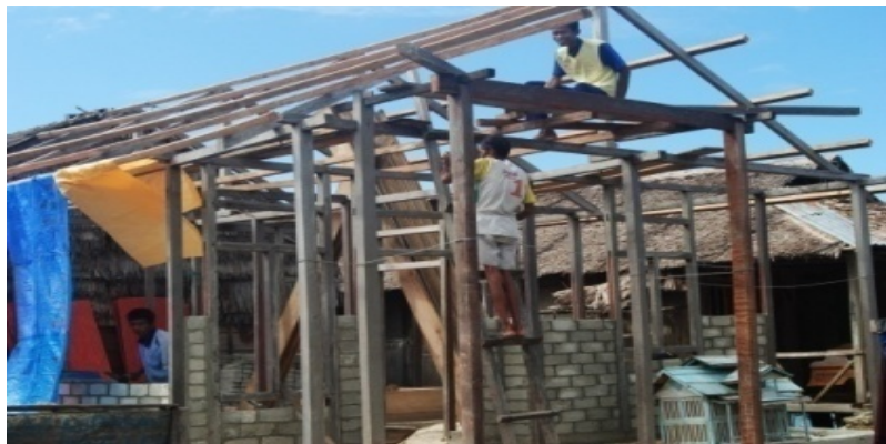
Figure 6. The frame of the building is made of wood with a hood frame. Source: Researchers' recorded images in 2009.
