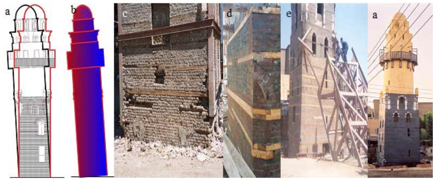
Figure 9. Stabilization the tendencies of the Esna minaret (a, b) architectural documentation (c) the base of the minaret after its tendencies and suffered many problems of damage (d) consolidation of the minaret from the outside by replacement of damaged elements, completion of missed parts and re stitching by wooden beams (e) removal of the steel works after completion of the repair work (f) minaret after restoration and stabilization of tendencies.
