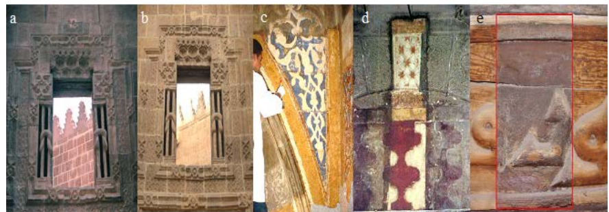
Figure 13. Different applications for the cleaning process (a, b) the upper part of the entrance of Hassan Pasha Taher Complex is characterized by the hollow sculpture of columns (c, d) cleaning of the color composition elements in the Sabil of Ashraf Qaitbay in Sayda Zeinab (e) clean a wood written carving tape.
