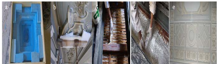
Figure 7. Stages of re construction of the back-support holder from GRP, (a, b) front protection work (c, d) implementation back support holder from GRP (e) decorative ceiling after reinforcement and removal protective layers.
