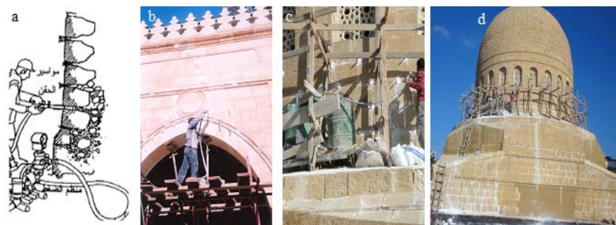
Figure 4. Various applications for injection work in reinforcing the internal fillings and filling gaps in the archaeological buildings (a) Sketch showing injection technique (b) Injection in the arches of the mosque Sayda Soukayna (c, d) Injection for re bonding of Internal filling dome of Ebrahim El Dousouky.
