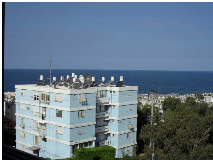
Figure 12. A house in Haifa, Israel, with water-boiling tanks on the roof. Photograph by the author.
