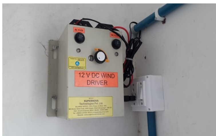
Figure 12. Variac for external 12V DC Motor.
