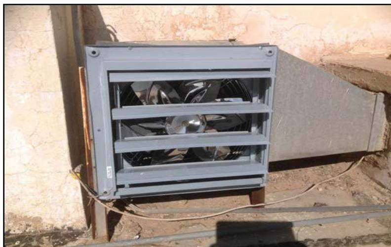
**Figure 9.** A set of fans have been installed at the end of the ducts.
