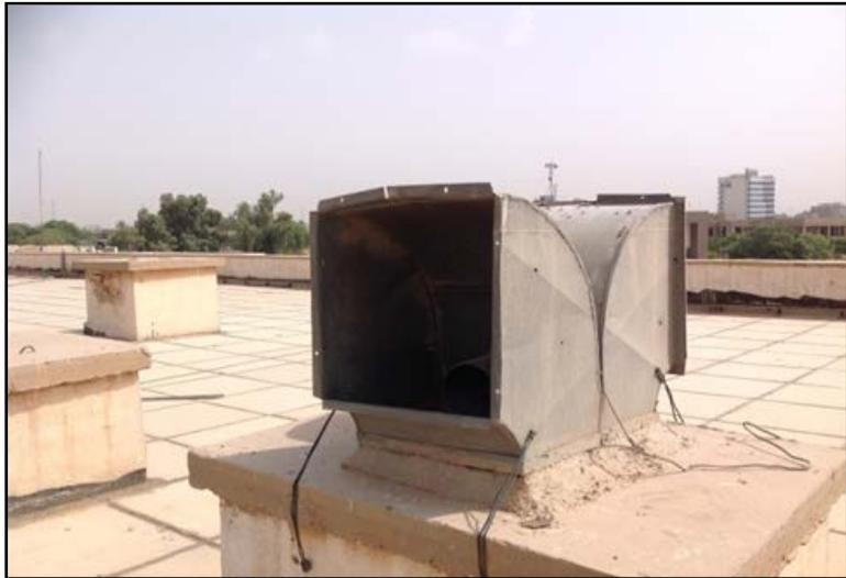
**Figure 4.** A duct which was not fitted with a barrier.
