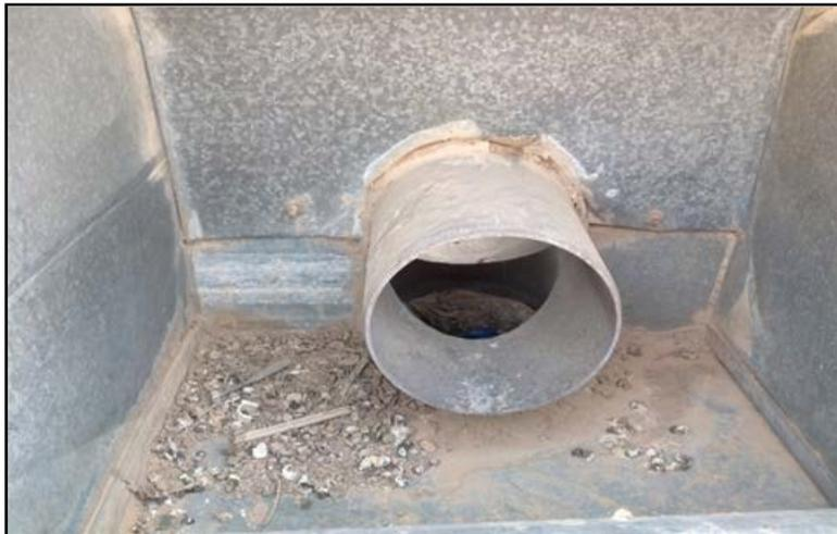
**Figure 5.** Another duct not fitted with a barrier.
