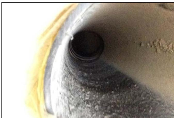
**Figure 1.** A white substance precipitated onto the internal surface of the ductwork.
