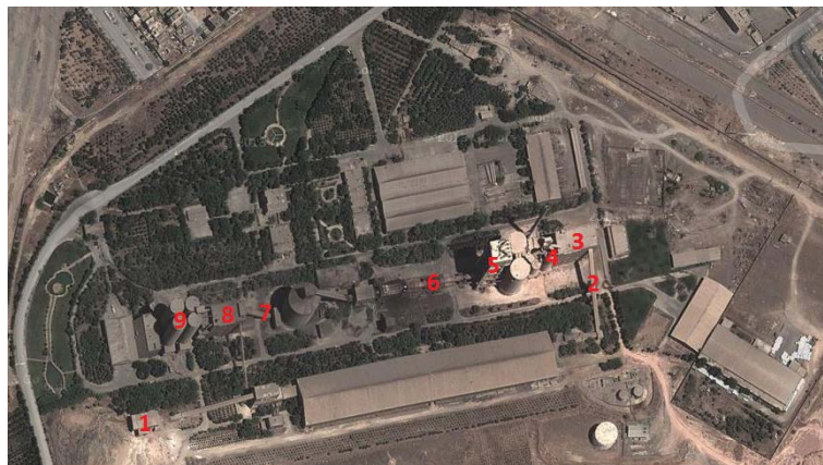
Figure 2. Top view of Tehran cement plant with tagged SPL measuring areas.
