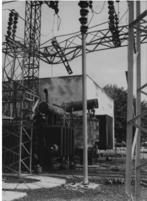
**Figure 2.** Collapse of overhead bus due to a fire.
