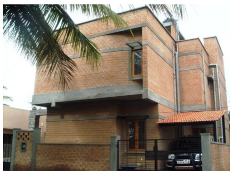
Figure 15. Residence constructed with Stabilised Mud Block.
