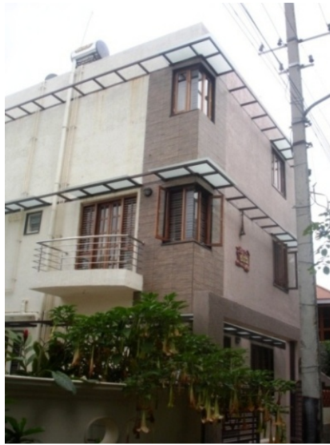
Figure 16. Residence constructed with Hollow concrete block.
