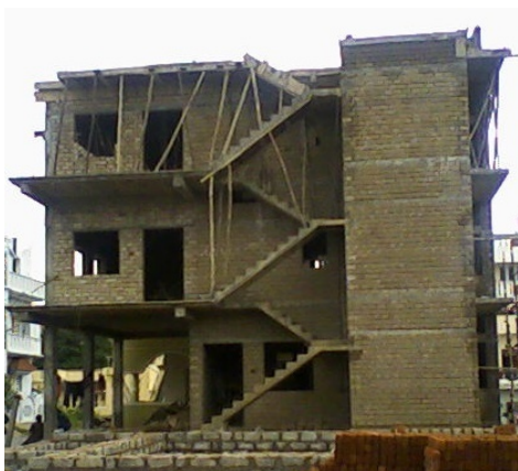
Figure 14. Residence under construction with PLB system.
