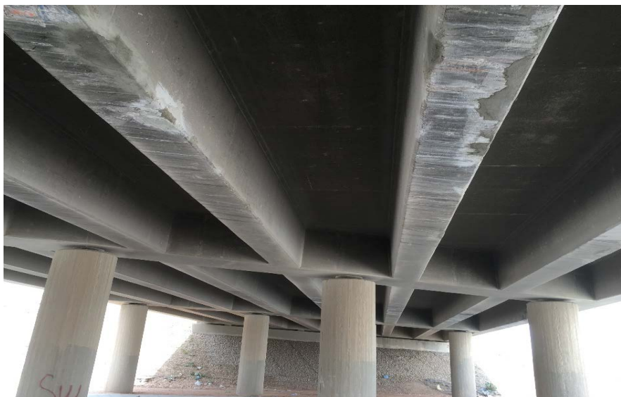
Figure 1. Al-Fahs bridge side view and lower deck view, respectively, (Riyadh, KSA).
