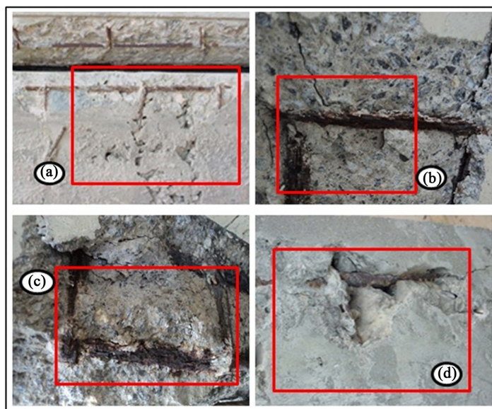
Figure 9. Example of corrosion in reinforcing steel.
