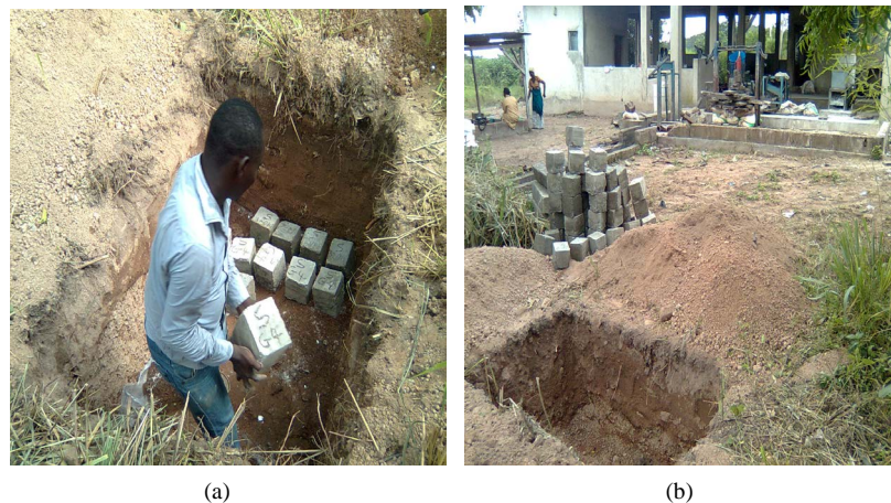
Figure 2. Excavated pits (a) natural unpolluted soil and (b) cyanide contaminated soil near cassava milling and processing site.
