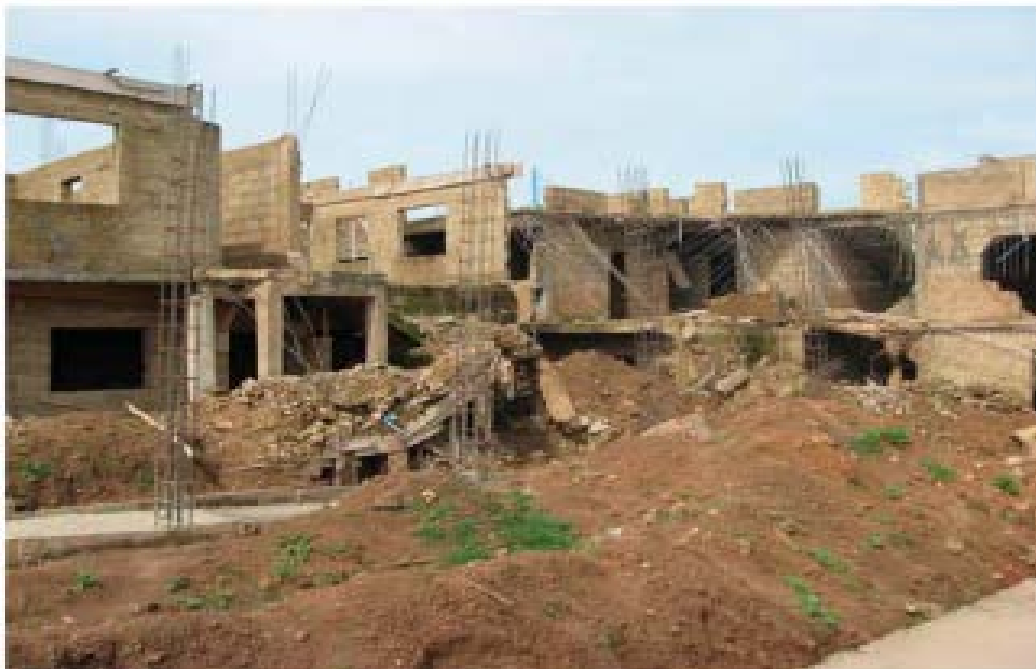
Figure 1. Collapsed part of the building.
