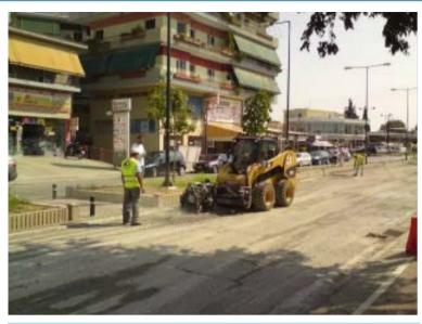
Figure 2. Removal of the old surface and cleaning at Vasilikon Street.
