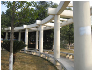
Figure 10. A local opened corridor.
