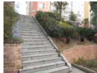
Figure 3. There are some steps but has no ramp besides.
