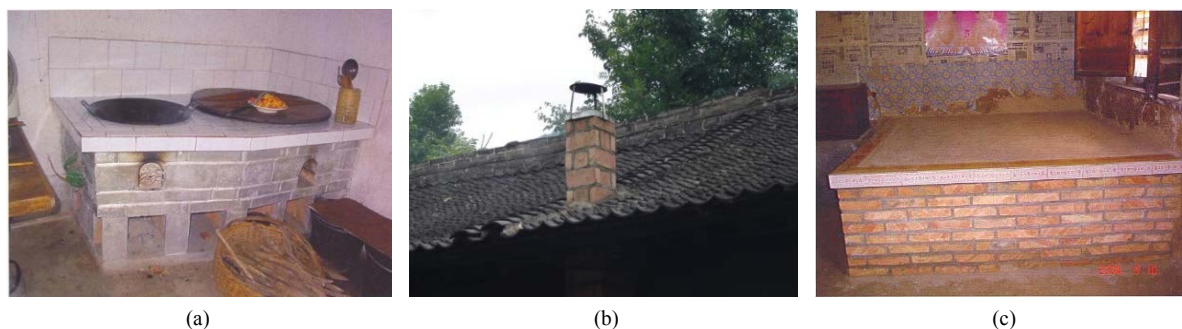
Figure 2. Improved stoves used by the households in the study area after the intervention. The improved stoves with a chimney that were used for the intervention (a) and (b) were specifically designed for the local residents. The improved stove was connected to a heating bed (called Kang as shown in (c)).
