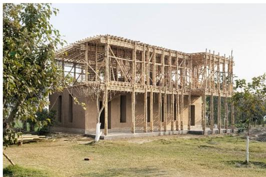
**Figure 2.** School built using local corn cobs and bamboo, Jar Maulwi, Pakistan.
