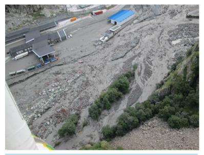
Figure 12. Damaged customs checkpoint building.
