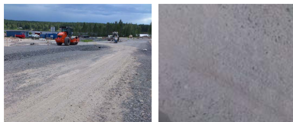
Figure 3. The unpaved road in Björnsby and the road surface.
