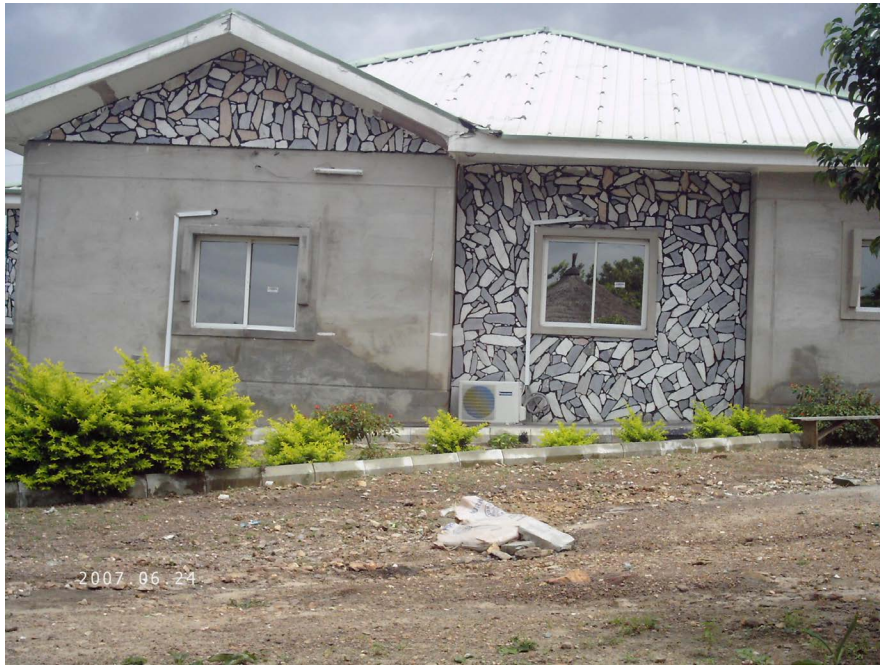
Figure 5. Use of marble for decoration at a house in the study area.
