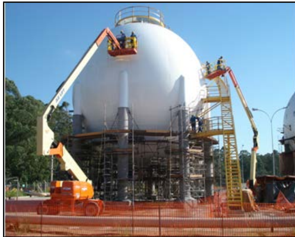
Figure 5. Application of finishing paint.
