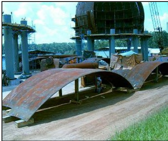
Figure 1. Industrial assembly of the sphere modules without paint application.
