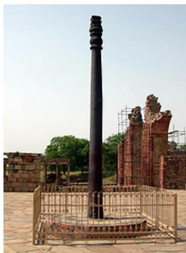
**Figure 1.** The iron pillar of Delhi, India [Chemical composition: 0.15% carbon, 0.25% phosphorus, 0.005% sulfur, 0.05% silicon, 0.02% nitrogen, 0.05% manganese, 0.03% copper, 0.05% nickel, and balance iron] [7].
