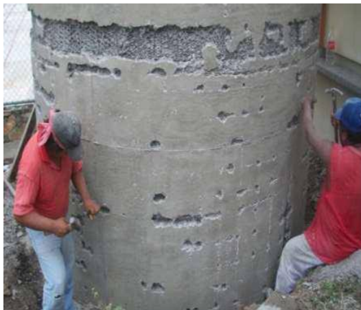
Photo 5. Constructive process, exterior finish [24].
