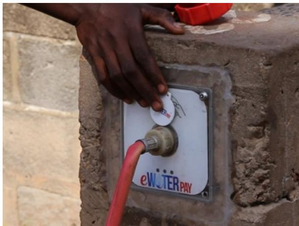
**Figure 1.** e-Tap and token in contact releasing water.
