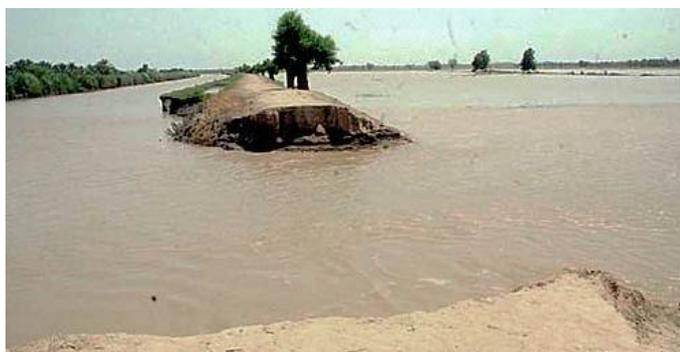
**Figure 2.** View of breach along Mir Wah Canal, Sindh [11].
