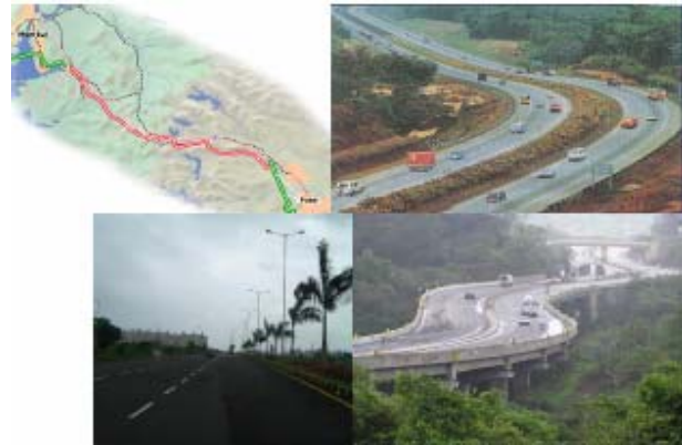
Figure 14. Scenario of mumbai-pune highway road.
