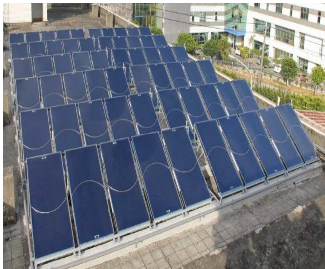
Figure 1. Solar water heater for sterilization.
