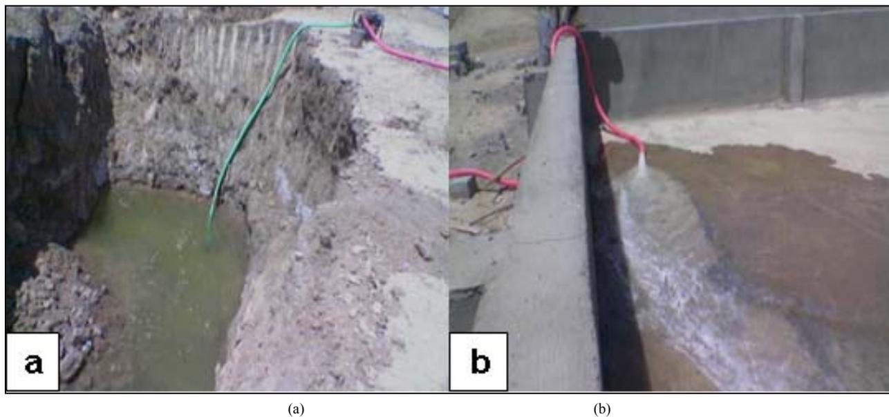
Figure 10. Illustration of (a) the nature of digging shallow wells excavated in the area near the constructed pond; and (b) the water pumped into the pond and water accumulated in the pond for evaporation.
