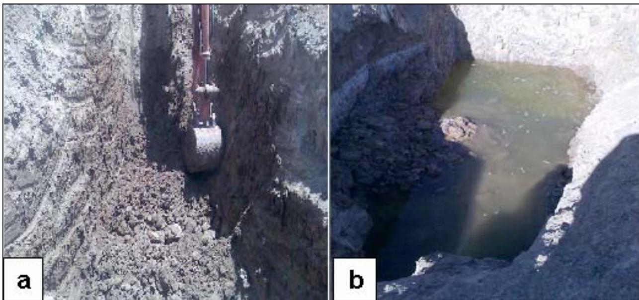
Figure 9. (a) Hole digging and (b) Water accumulation in the digged hole.
