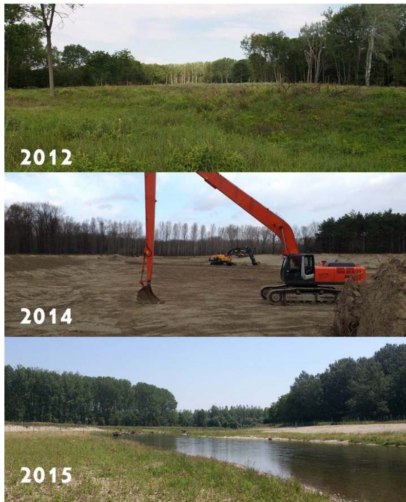
Figure 1. Construction section No.1 over the course of work in 2012, 2014 und 2015.
