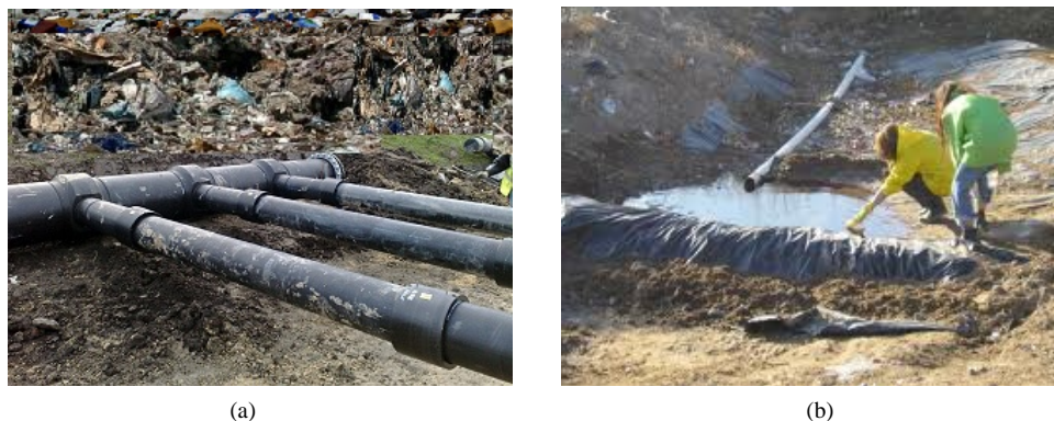
Figure 7. Examples of remediation: (a) drainage pipes placement and (b) impermeable thin substrate.
