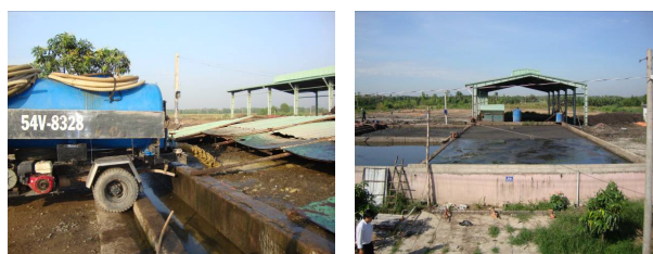
Figure 5. Transportation and treatment facilities (producing compost fertilizer) of sludge generated from septic tanks at Hoa Binh plant (Da Phuoc Waste treatment complex—Binh Chanh).
