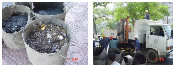
Figure 1. Sludge from dredging of wastewater drainage network.
