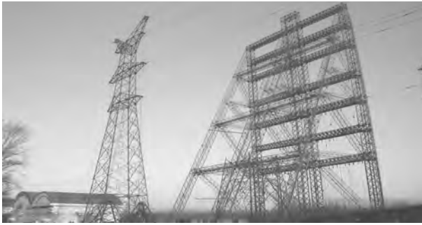
Figure 9. Test tower and loading tower
