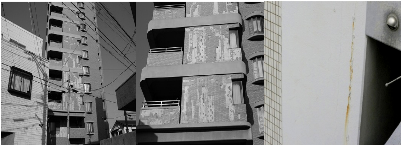
Figure 7. The defective parts (concrete cracks) of the outer walls of buildings.
