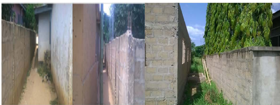
Figure 3. The narrow spaces in-between new residential buildings.
