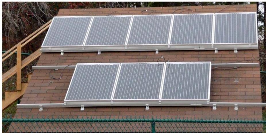
**Figure 3.** Photo of Trial 1. Upper array shingle flush 5 modules, lower array shingle flush 3 modules. (Refer to Table 1 for details).
