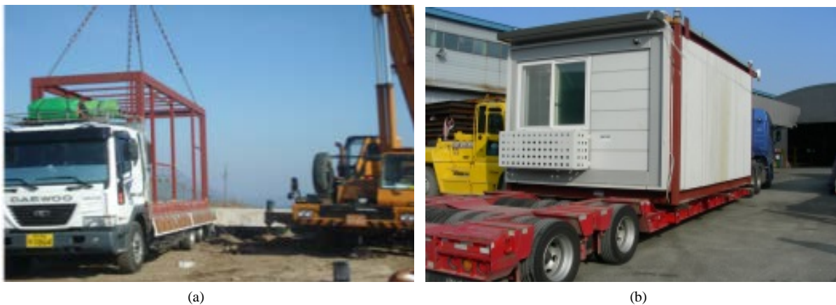
Figure 1. Unit modules' prefabrication percentage [6]. (a) 40% - 50%; (b) 80% - 90%.
