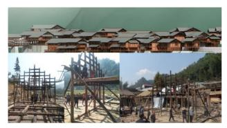
Figure 15. Directing Tujia people to build new stilted buildings using authentic traditional techniques picture by Kui Zhao, 2010.
