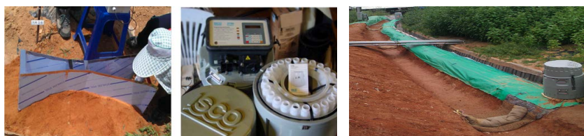
Figure 4. Installation of parshall flume and automatic sampler (left) and hybrid BMP within a ditch (right).
