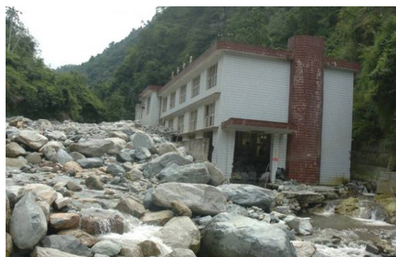
Figure 6. Outburst debris flow buried the Heiqiao power station.
