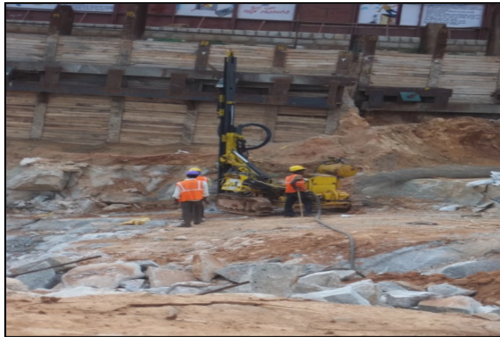
Figure 2. A view of drilling operation at excavation site.
