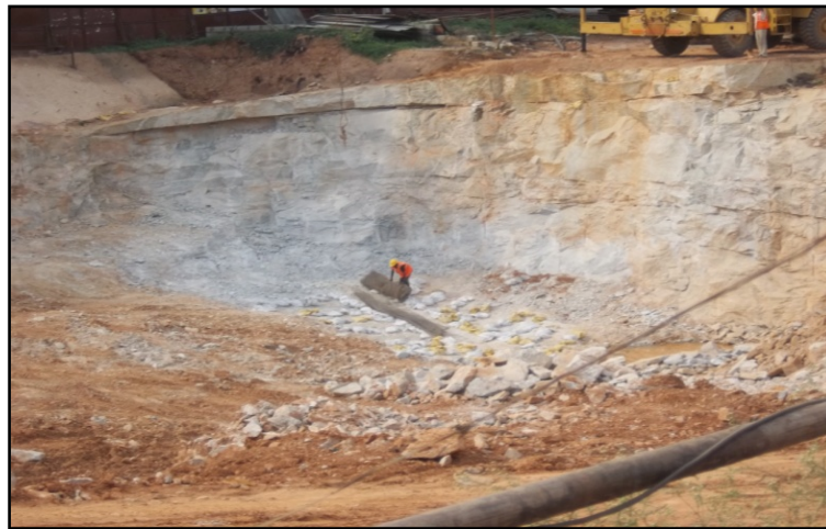
Figure 3. A view of blast site.
