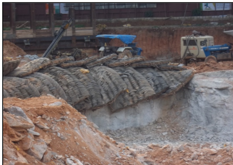
Figure 4. Muffling arrangement on blast area.
