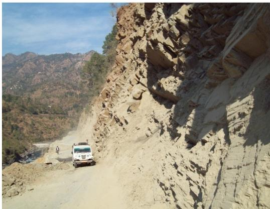
**Figure 3. A cut slope section of the study area showing negative slope with 3 sets of joint.**
