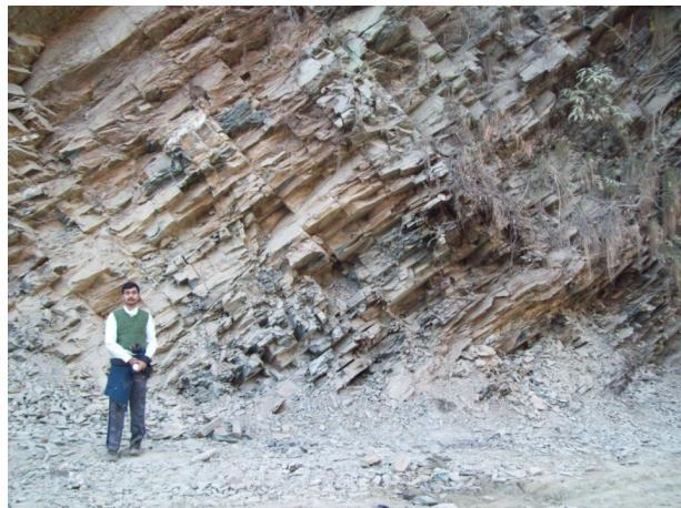
**Figure 5. Very closed space jointed phyllitic rock with higher persistency.**
