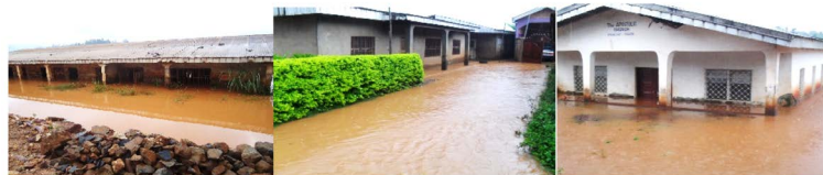
Figure 5. Houses affected by floods at below Foncha and Ndamukong. Source: Fieldwork 08/09/2014.
