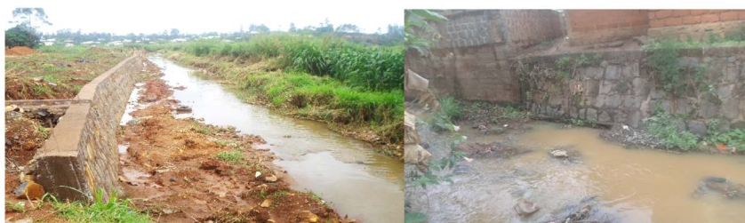
Figure 9. Channel straightening and embankment. Source: Fieldwork, 03/27/2015.
