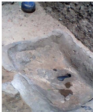
Picture 3. A device of management of gray wastewater from 1987 connected to a gutter at Maradaoua district.
