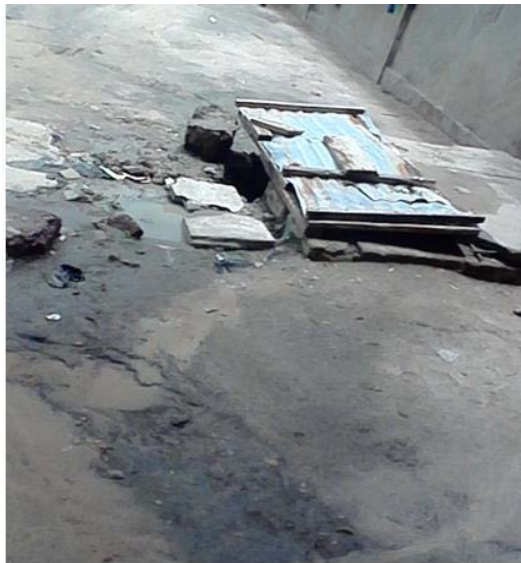
Picture 8. Septic shabby spilling its overflow downstream (Dan Goulbi district).
