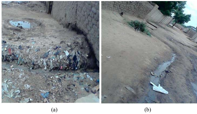
Picture 5. Disposal systems gray waste water of households connected to public roads in the town of Maradi ((a) Yandaka district; (b) Bourja district).
