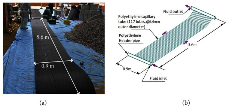
**Figure 4.** Capillary mat heat exchanger being prepared for installation (a) and its schematic description (b).
